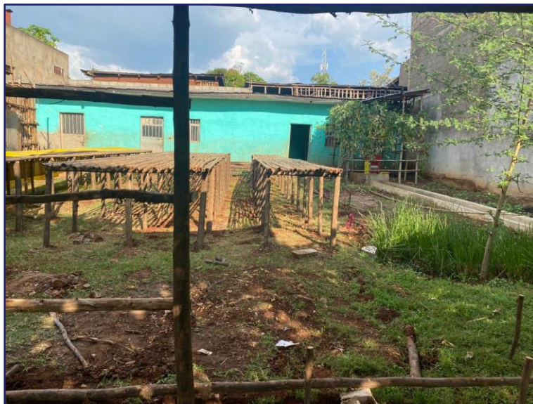
Dilla experiment site under construction at the TNS office.
