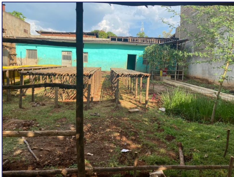
Dilla experiment site under construction at the TechnoServe office.
